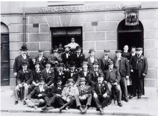
8 | The Gas Fitters Arms, Tidy Street. Image courtesy of The Regency Society. For further details about this photograph, see: http://www.regencysociety-jamesgray.com
