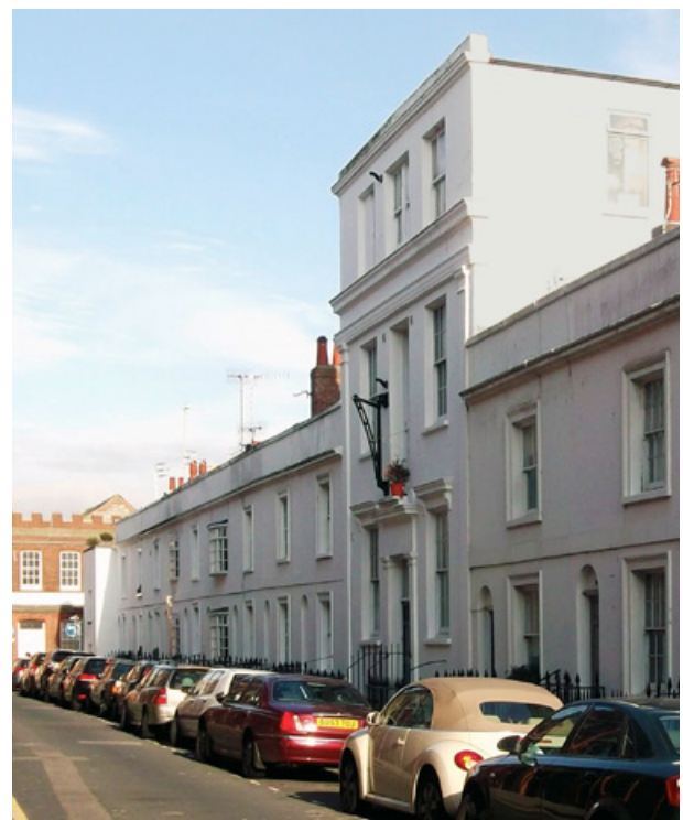
8 | A contemporary photograph of Robert Street, the two-stories of the original Jireh Chapel can be seen, beneath the third storey added in 1898
