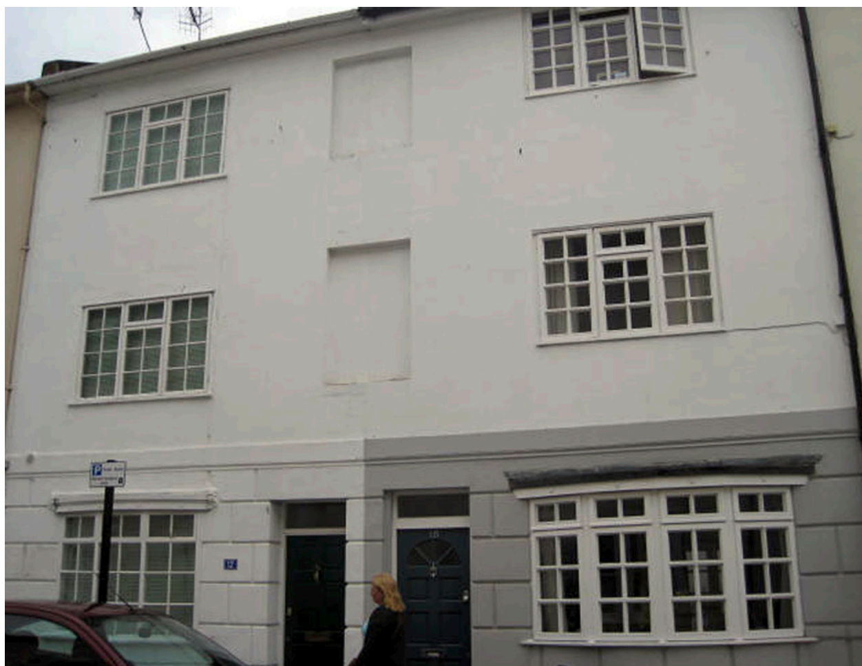
7 | Numbers 17 and 18 as they are today with the old shop fronts having been rebuilt. Image courtesy of Catherine Page
