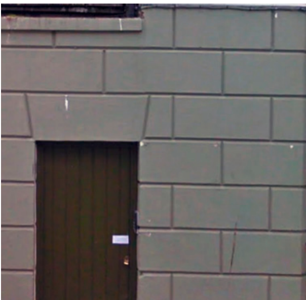
4 | Typical rusticated finish to elevations in Over Street
